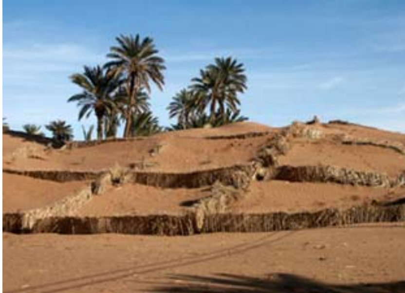
Figure 7.6-2: Stabilization of sand dunes in Souss-Massa
