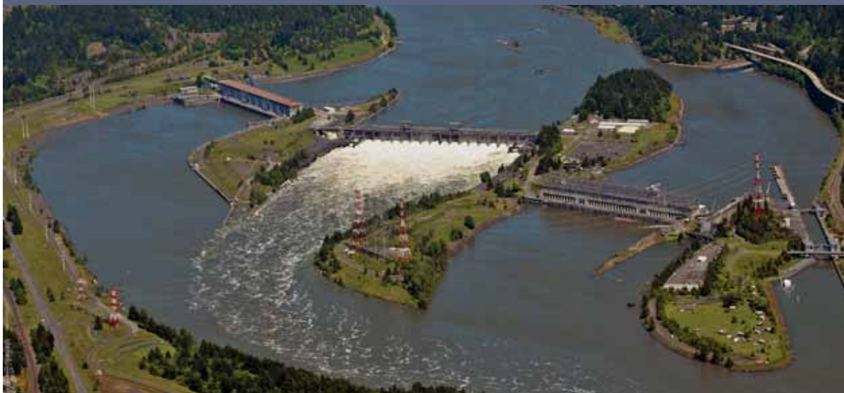
Bonneville Dam on the Columbia River near Cascade Locks, Ore
