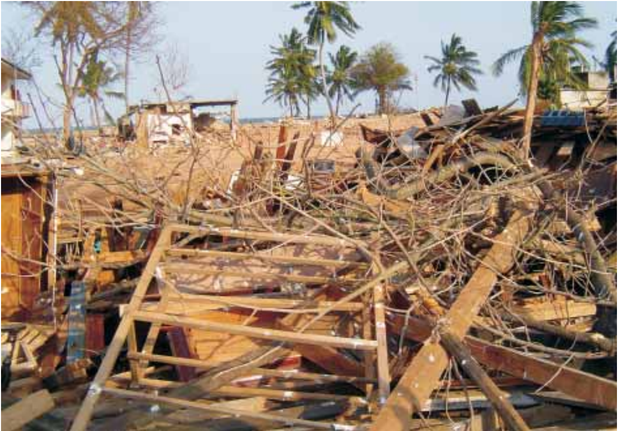
Managing the tangled mass of debris was an immediate challenge after the tsunami. Credit: Dr J.Samarakoon.
