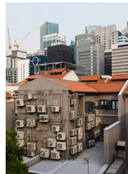
Air-conditioning units on a house in Singapore, 2013.
