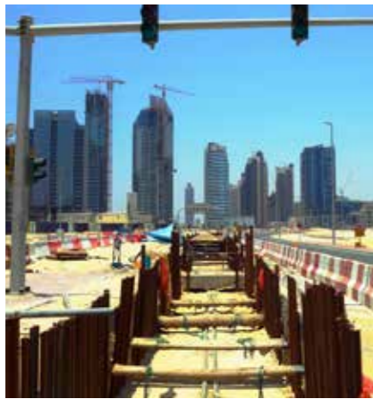
Laying district cooling pipes in Dubai, UAE.
