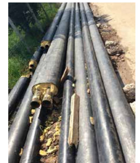
New city development in China (top). Pre-insulated district heat pipe in Botosani, Romania (bottom).
