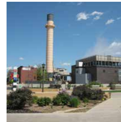
Renewable CHP plants, such as this wood-fired plant in St. Paul, USA, could provide the primary energy efficiency improvements and renewable heat that could count towards an improved efficiency label for a building.
