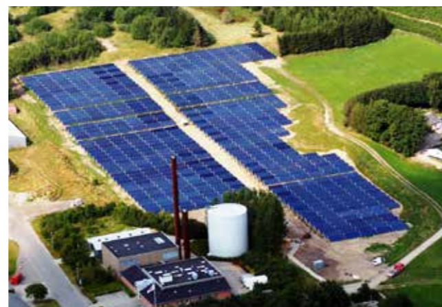
A large solar thermal plant with heat storage connects to a district heating network in Brødstrup, Denmark.
