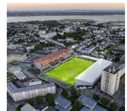
Oslo, Norway (top). Stade Francis le Blé in Brest (bottom). Connecting stadiums, leisure centres, hospitals and other anchor loads diversifies the load, making the district energy system more efficient.
