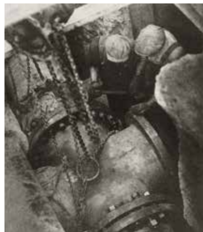
Installing a two-metre-diameter steam pipe for district heating in New York in the early 20th century (left).
