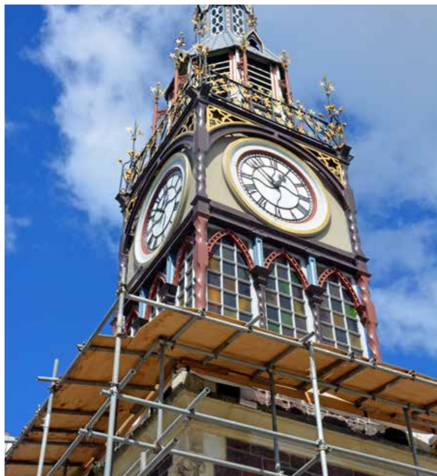
Restoring Christchurch's landmark Diamond Jubilee Clock Tower after the 2011 earthquake.
