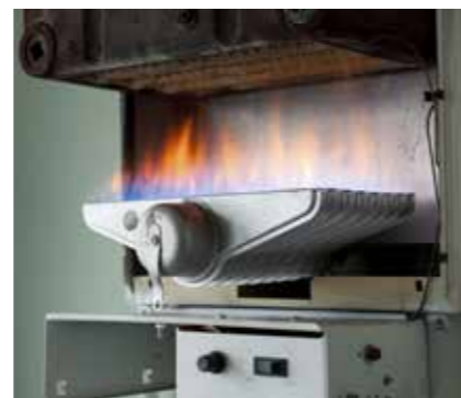
Individual air-conditioning units (top) and gas boilers (bottom) are just two of the technologies that district energy can replace.
