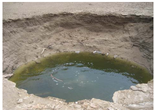
Sink hole caused by low water levels in the Dead Sea. Photo credit: OSU Geo Club.
