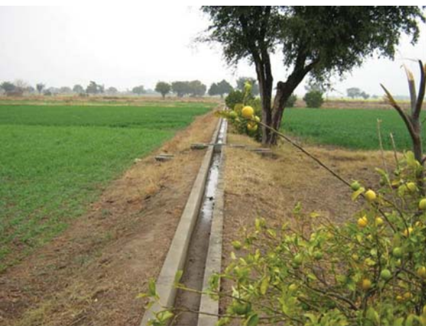
Drain for irrigation water drawn from wells near Bhaun, Pakistan, Indus River basin. Photo credit: Syed Usman Ali, via Wikimedia Commons.
