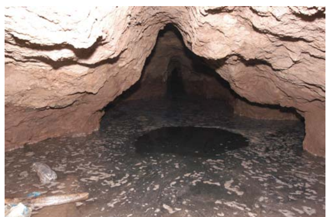
(from top) Aerial view of qanat system of Bam, Iran; descending into qanat to perform maintenance; cleaning out the qanat; view of inside the qanat. This ancient form of water infrastructure is still widely used in arid and semi-arid regions to provide irrigation water and water for household usage. Water from aquifers or rivers is channeled through gently sloping subterranean canals. Photo credits: Babak Sedighi.
