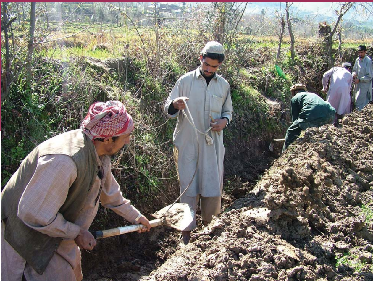
Villagers and farmers work together to clear this 3.5-km-long irrigation canal in the village of Sir Ajmaira, in Pakistan's northern Battagram District. Once cleared, it will irrigate 375 acres of wheat, rice, and vegetables. Photo credit: Kaukab Jhumra Smith, USAID.
