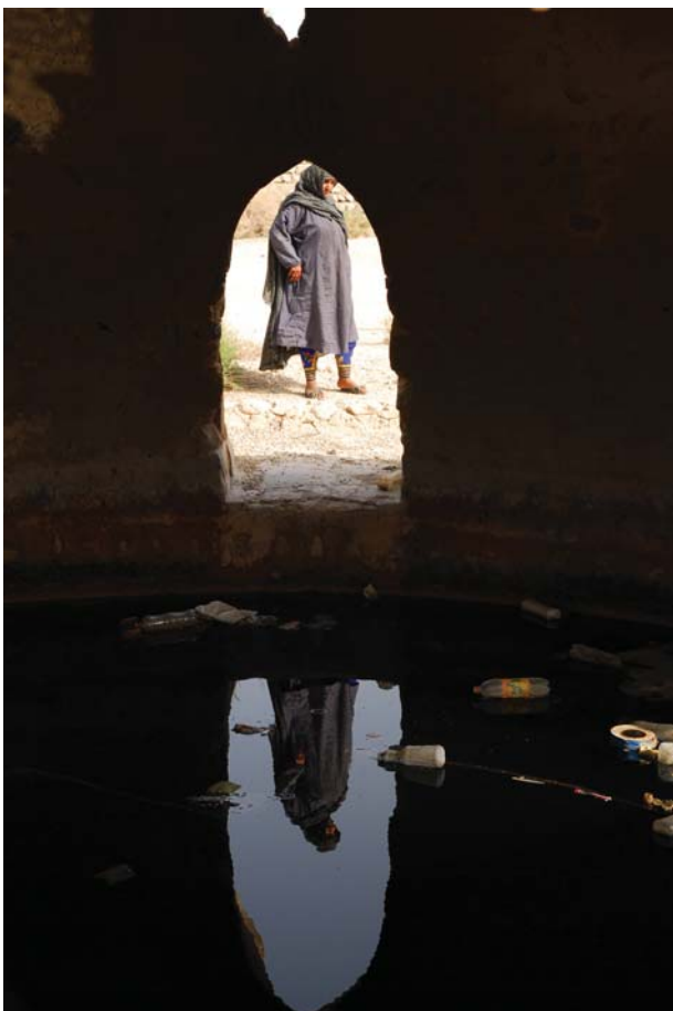
Reflection in the debris-filled water of a birkeh; this ancient form of infrastructure is used to collect and store water for community use in southern Iran and other arid regions. Photo credit: Babak Sedighi.
