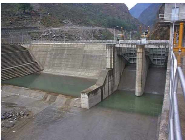
Bhote Koshi hydropower project, a 36-megawatt powerhouse in a remote area of Nepal, on the Bhote Koshi, a river fed by snowmelt from the Himalaya Range. Photo credit: USAID.
