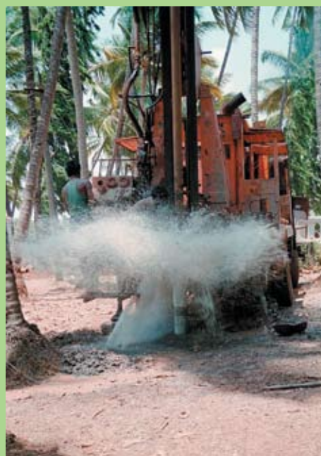
SUCCESSFUL WATER DRILLING, GOA, INDIA
