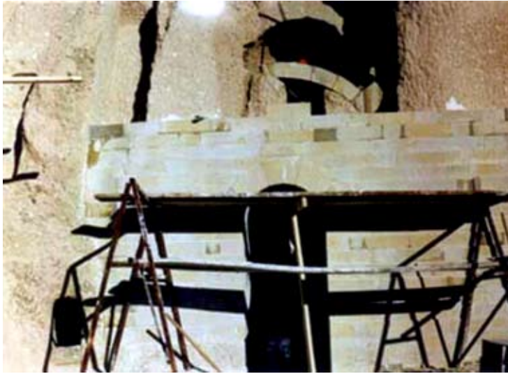
EXTERIOR VIEW OF THE RESTORATION
