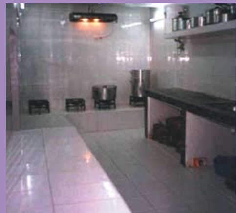
KITCHEN AFTER RENOVATION, HOTEL MOUNIA, FES, MOROCCO
