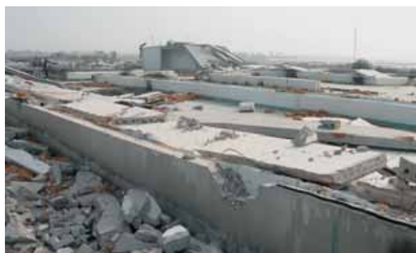
The primary problem in Kfar Darom is rubble removal
