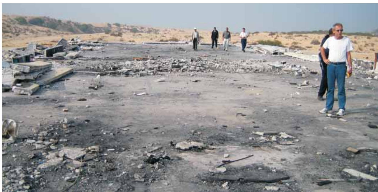
The concrete slab on location A in Rafiah Yam
