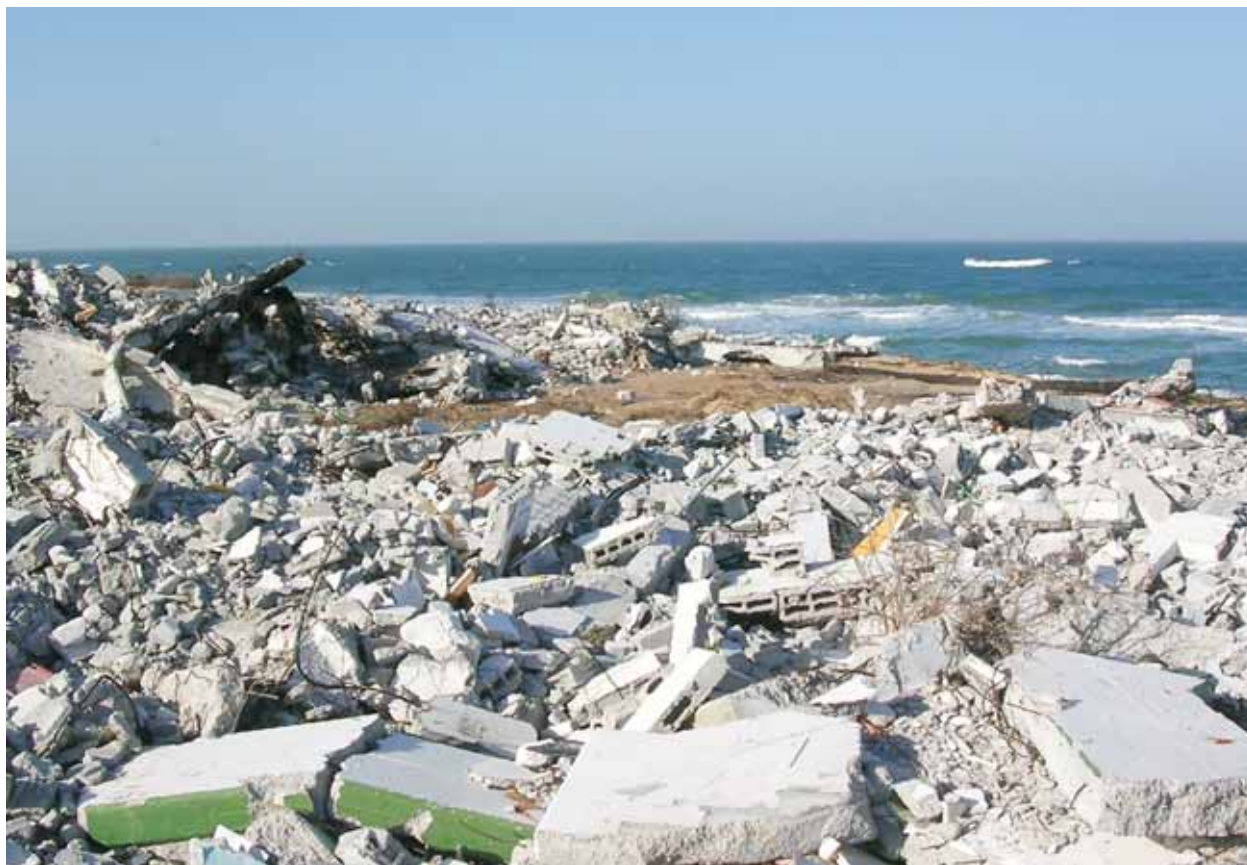
Rubble at Gaza Beaches site
