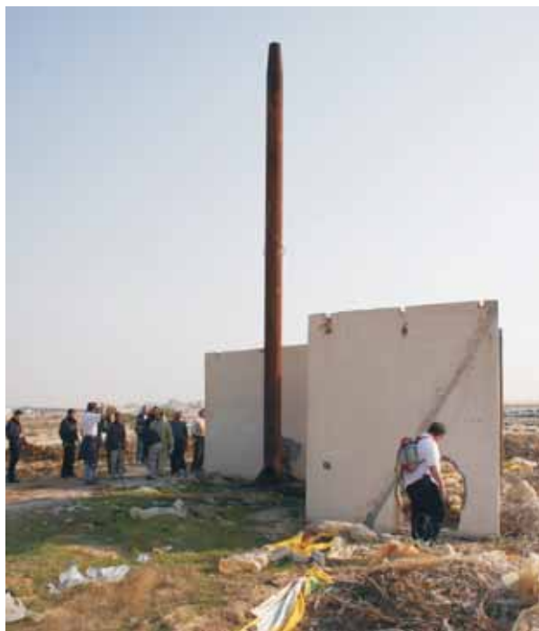
A view of the chimney to a unit in Gadid. Sampling illustrated elevated concentrations of pH and Nickel
