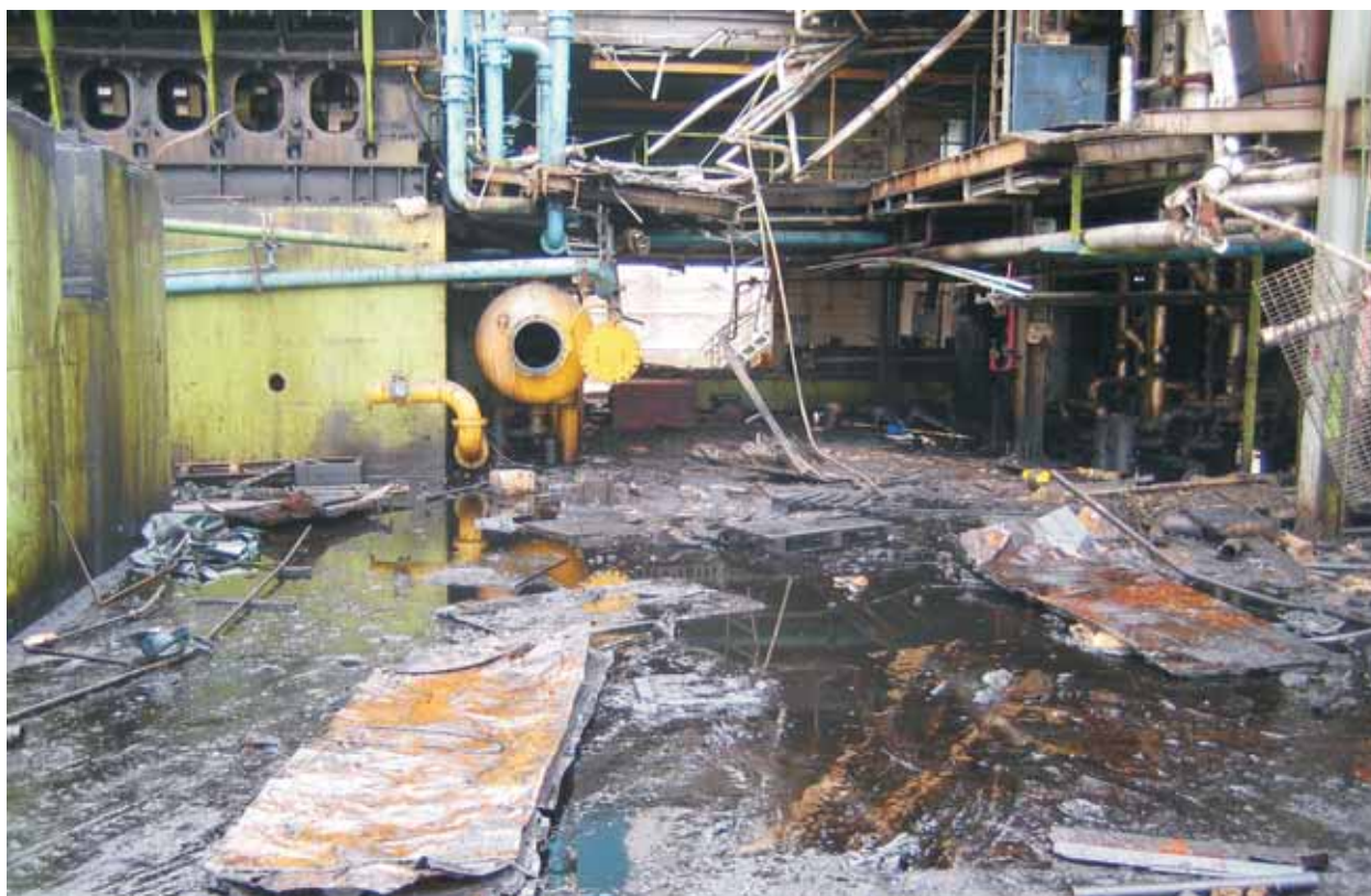
Spilled oils on location in Erez Industrial Estate
