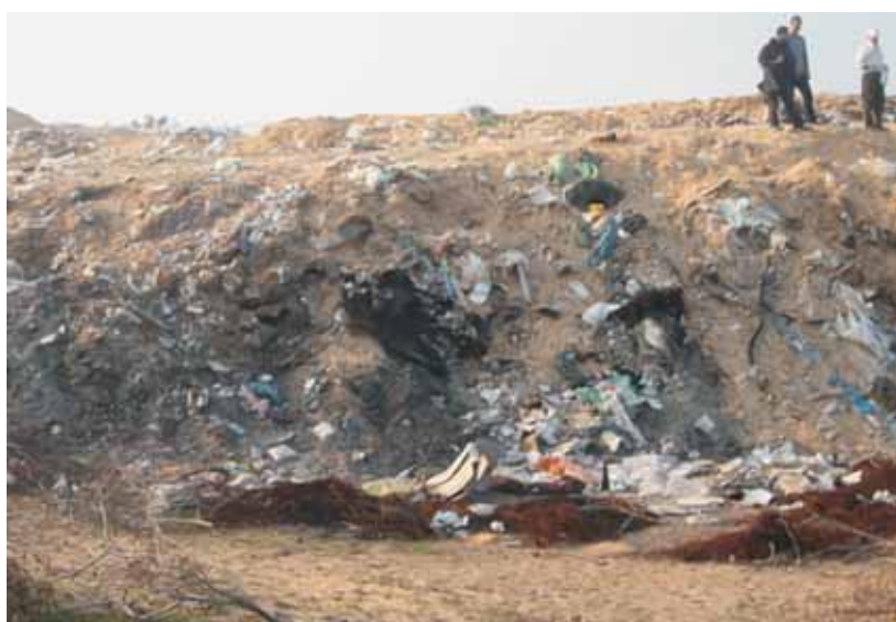
The exposed operational face of the waste disposal site at Kerem Atsama
