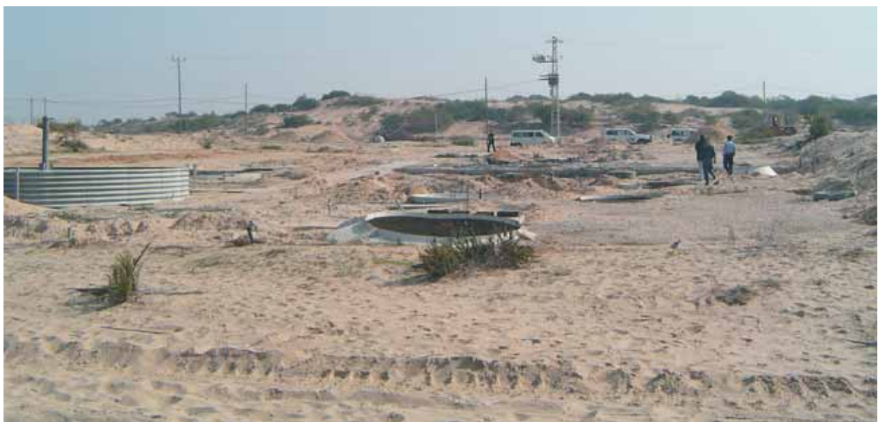
The derelict sewage treatment plant in Nieve Dkalim
