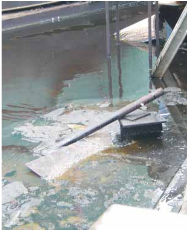
Spilled oil inside cemented isolation structure
