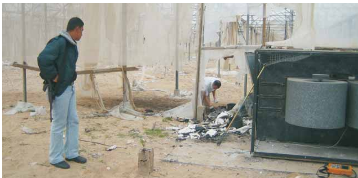
A greenhouse heating unit with localized oil spill in the background
