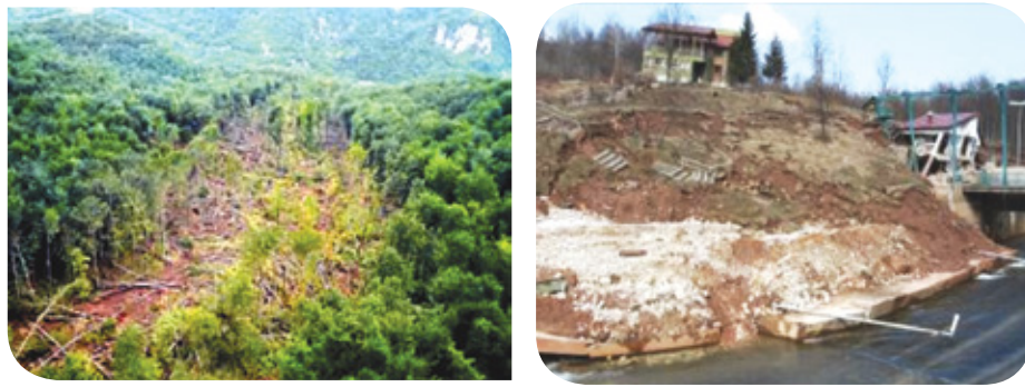
Figure 136: Massive landslide in Bogatići (2010) which destroyed a hydropower plant and part of the forest
