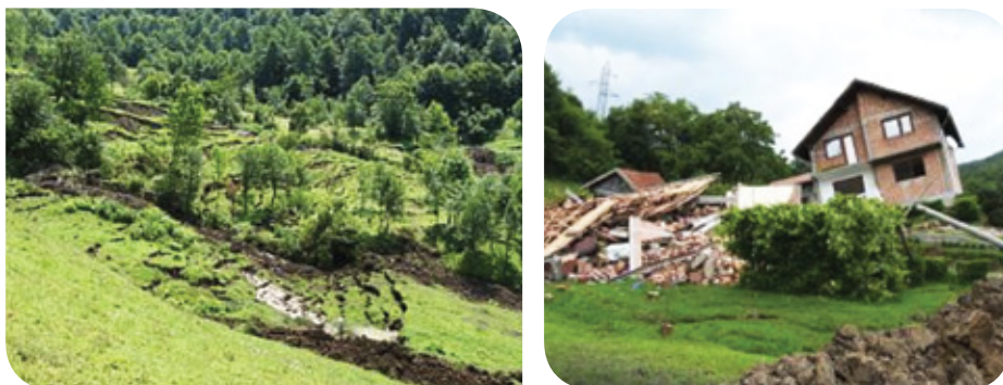
Figure 135: Landslide in Suljakovići (2010.) near Maglaj, that caused a total infrastructural destruction and environmental damage
