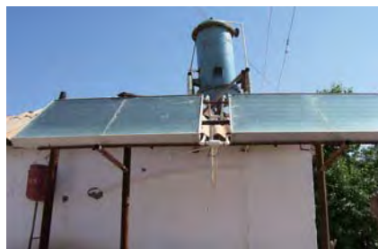
Solar-Thermo Panel Installation (exterior, shower premise, School Bahardock)
