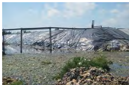
Methane transport pipes in Pontianak
