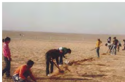
Youth excavating soil to lay pipes for irrigating farmland
