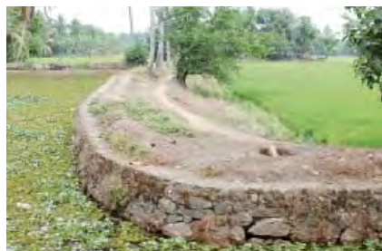
Ridge that protect paddy field from flooding
