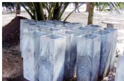
Biosand filter being constructed
