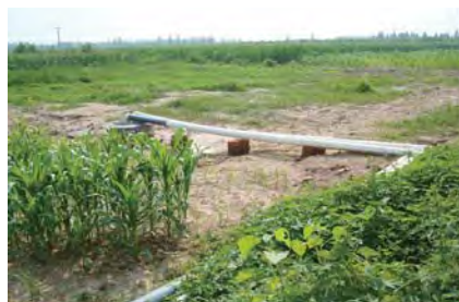
4-Pipes collecting polluted waters
