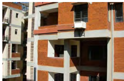
T-Zed apartment blocks showing projecting and receding massing creating shading for the lower floors
