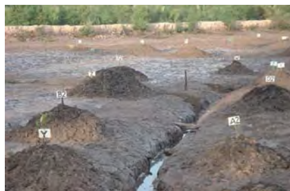
Pond land preparation work
