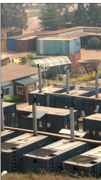
Diesel powered generators in Gikondo Valley in Kigali supplement the shortfall in the electricity supply from mainly hydropower sources that are still not able to meet the rising demand levels.
