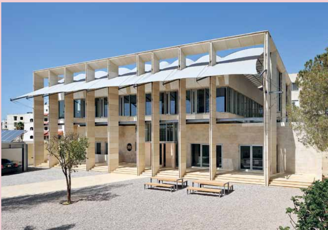
Front elevation with colonnade and shading. Solar hot water panels on the carport (left).
