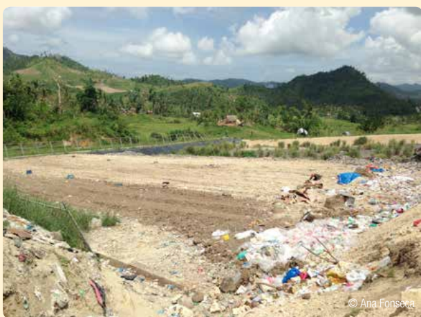
Active cell partially managed: waste compaction, daily cover and vents in place –during UNDP WMC intervention
