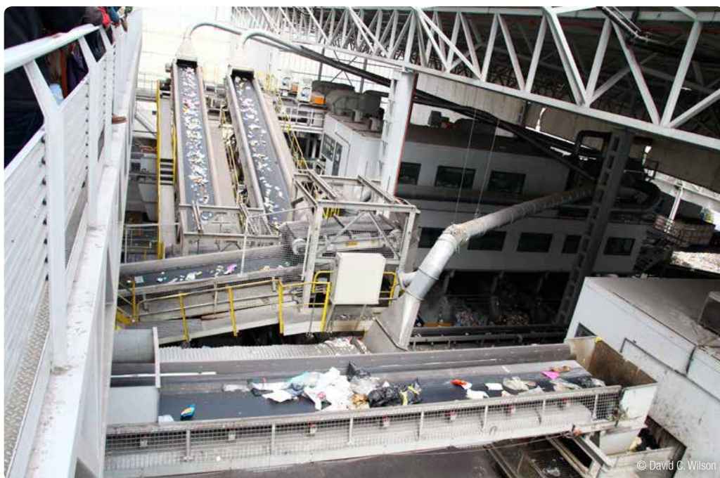
Separation of wastes in an MRF/MBT plant in Madrid, Spain
