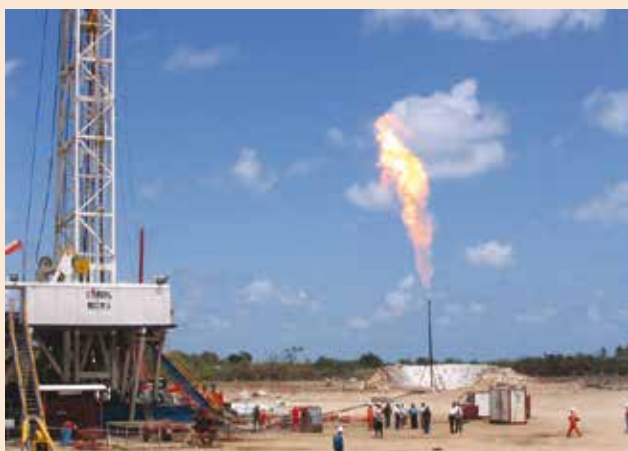
Testing a new methane gas well, Songo Songo Island, Tanzania. © Matthew D. Richmond.
