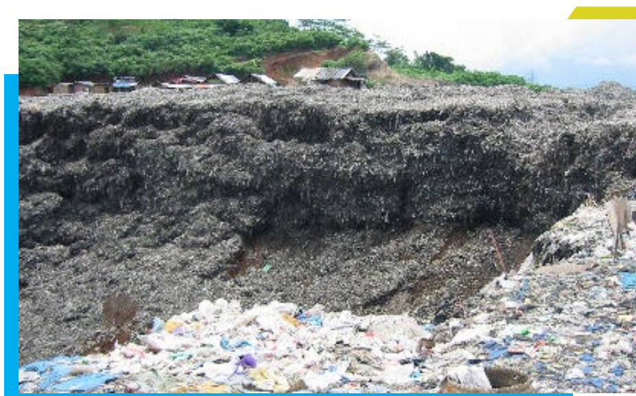
Figure 8: Slope crest of Leuwigajah dumpsite 59
