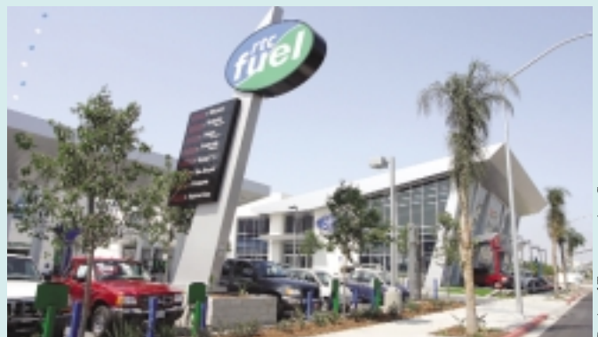
Regional Transportation Center
