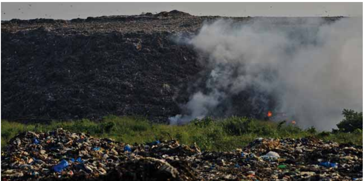
Fires are common in the existing landfill
