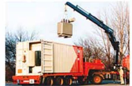
Picture 100: Loading of transformers
