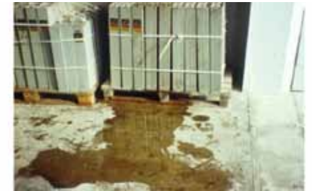
Picture 85: Bad example II (no tip trays)
