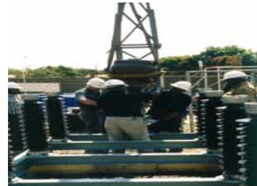
Picture 55: Dismantling of capacitor battery
