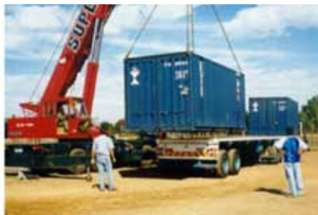
Picture 98: Lifting of containers to truck
