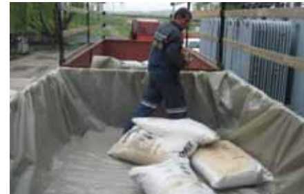
Picture 69: Preparation: transportation of PCB transformer
