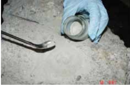
Picture 19: Sampling of concrete
