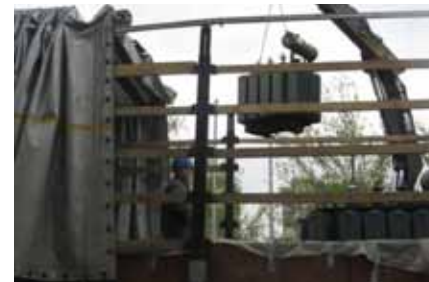
Picture 71: Loading of transformers
