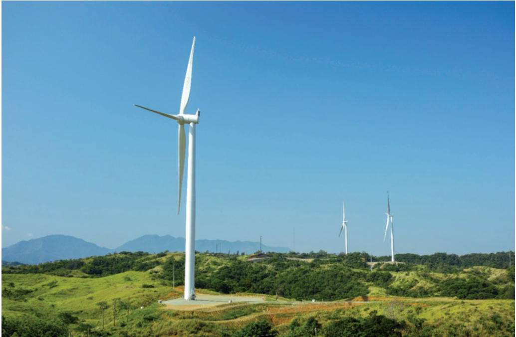
The 81 MW Caparispisan Wind Energy Facility. Photo courtesy of North Luzon Renewables/AC Energy
