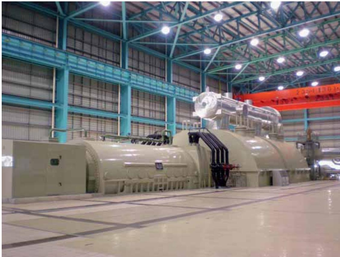
One of the ultra-supercritical generators at the Waigaoqiao Third Power Plant.
