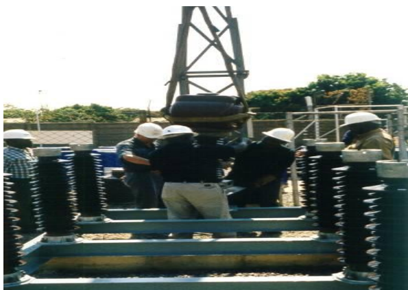
Picture 55: Dismantling of capacitor battery
