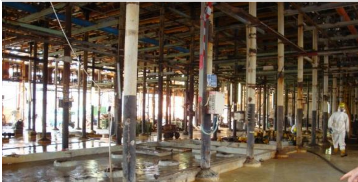
Floor of cell room regularly washed down
