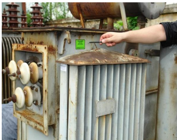
Picture 12: Affix labels while sampling and later final one
