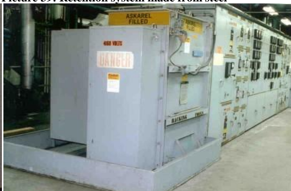
Picture 39: Retention system made from steel
