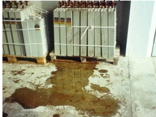
Picture 85: Bad example II (no tip trays)
