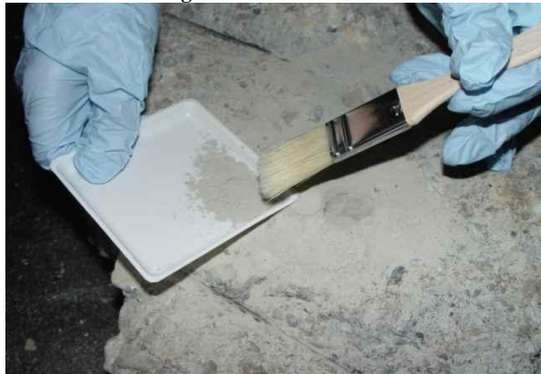
Picture 20: Cleaning of leftover dust
