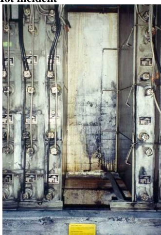
Picture 49: Hot incident
