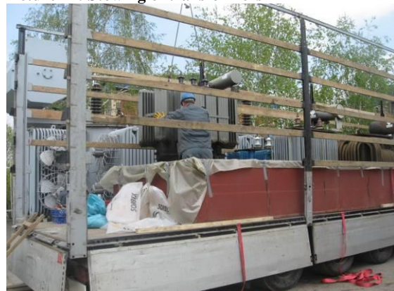
Picture 72: Stowing of transformers
