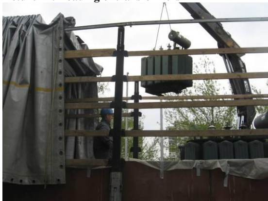
Picture 71: Loading of transformers
