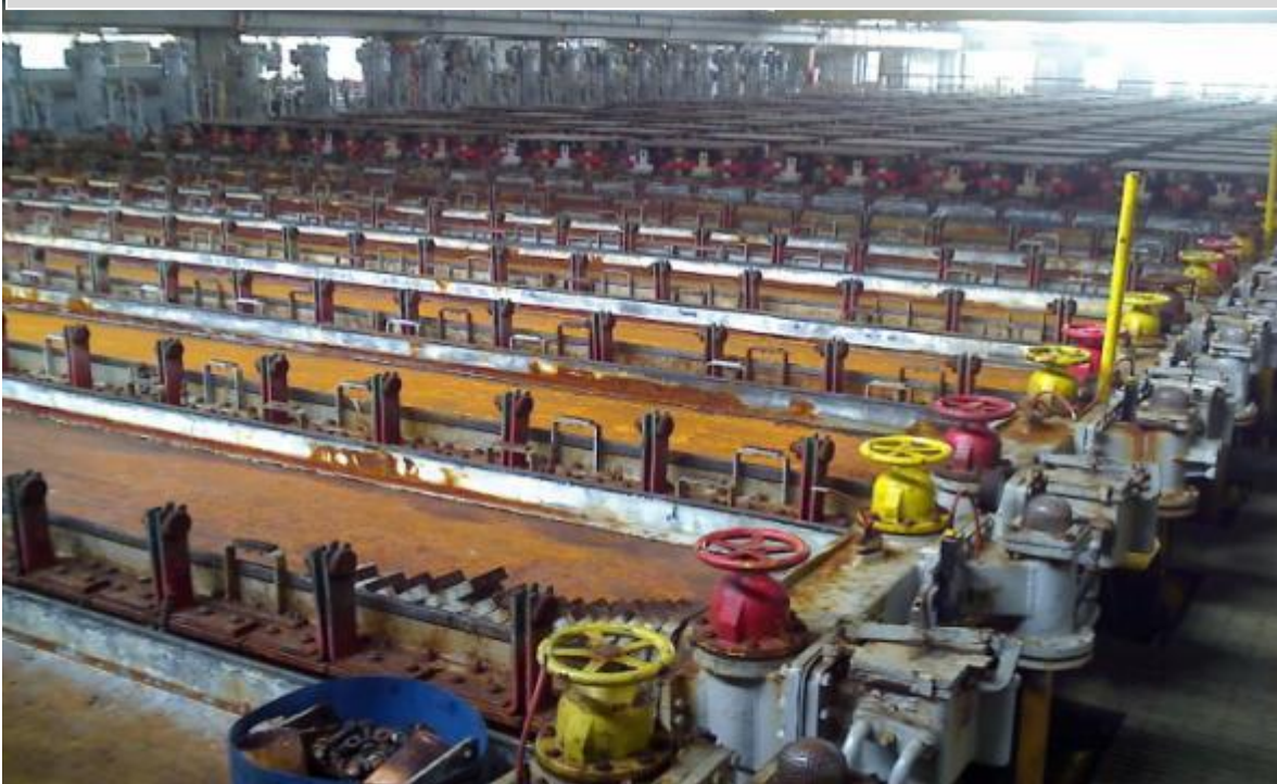
First stage of operations
