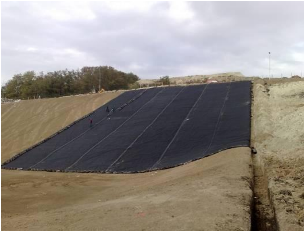
Fig. 35: Artificial barrier using HDPE foil for landfill
