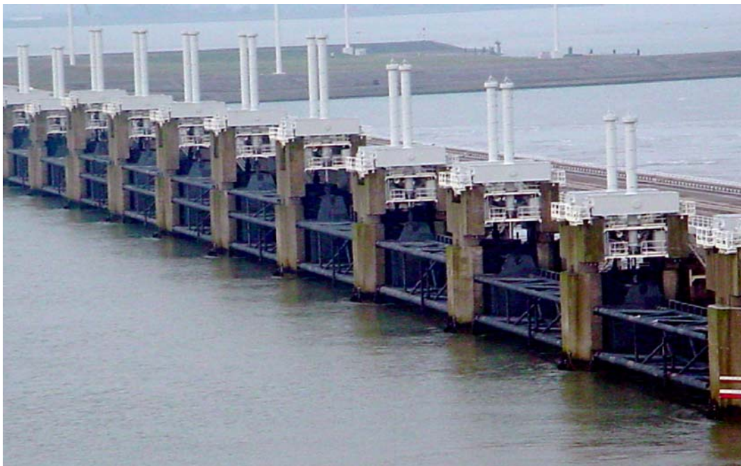
Fig. 3.4: Dams on the Oosterschelde protect the southern part of the Rhine-Meuse and Scheldt Deltas in the Netherlands against flooding. These dams were built in response to a major storm and flood event in 1953 in which over 2300 people were killed across the North Sea region. The dams have sluices through which tidal water freely move in and out to preserve the marine-estuarine ecosystem, but during major storms sluices are lowered. (Photo: James Syvitski).
