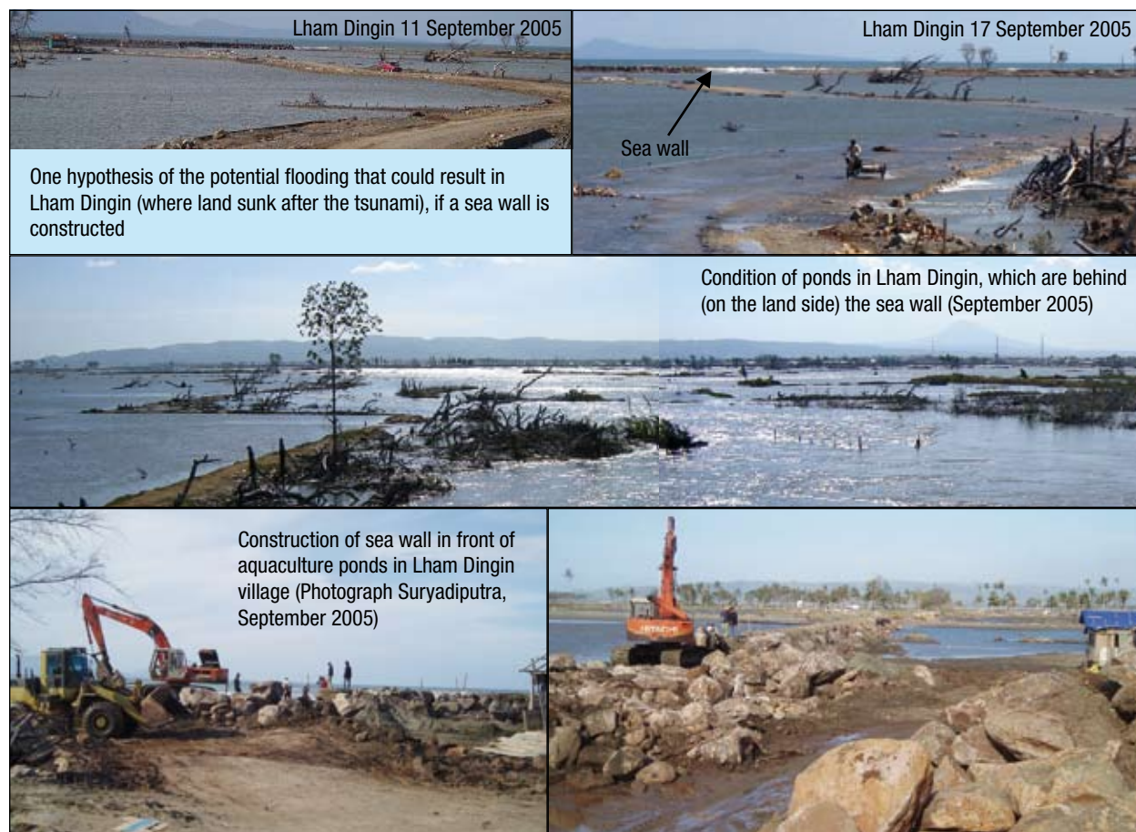
Figure 4.11. Lham Dingin flooded with sea and river water (Photograph WI-IP 11 & 17 September 2005)
