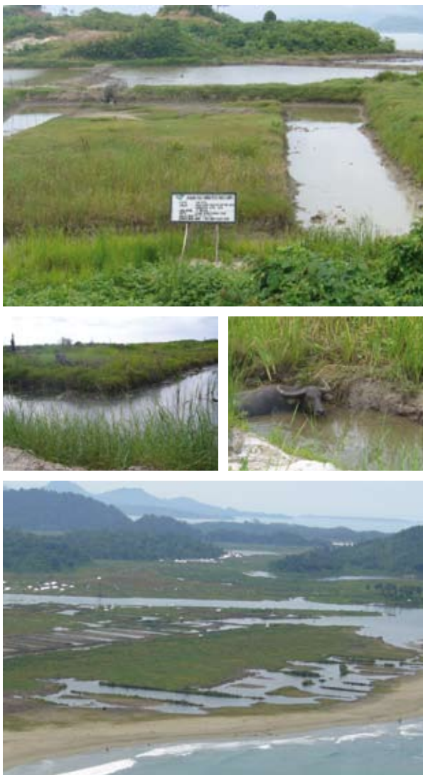
Figure 4.12 (Top, Middle left) Pond dikes and land (empty land in centre) where mangrove could be planted (these ponds are in Ceunamprong and Kareng Ateuh villages in Jaya subdistrict of Aceh Jaya district, and have been rehabilitated by BRR). (Middle right) One of these ponds has become little more than a buffalo wallow. (Bottom) Pond on Lhoong coast in danger of abrasion. Mangrove needs to be planted along the shore in front.
