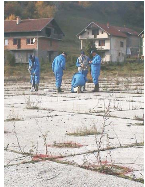
160 contamination points were found on this large concrete surface in the site's northwest corner
