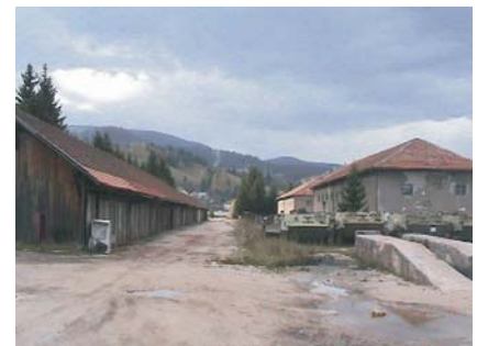
A westward view of the site
