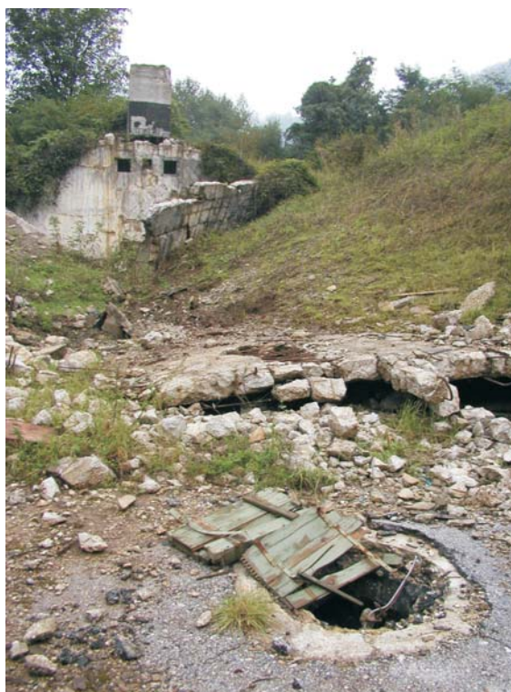
Storage bunkers were completely destroyed
