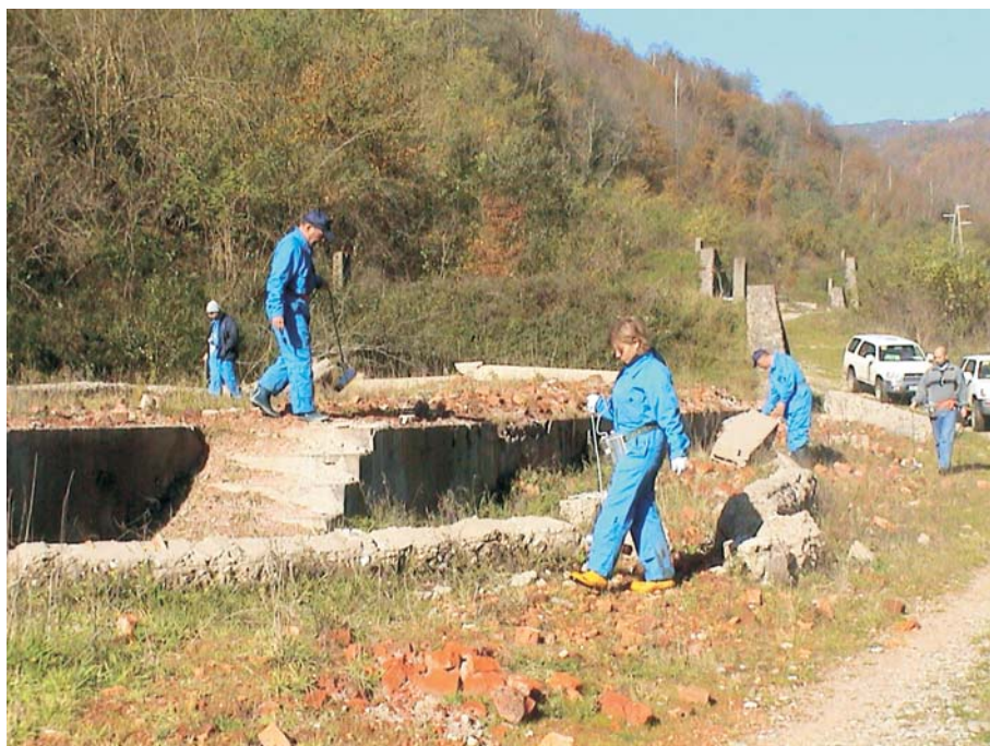
On-line and random survey techniques were used over hard surfaces in Ustikolina
