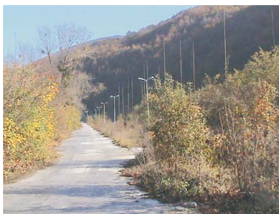
The many lightning rods throughout the site were used to prevent the live ammunition from being struck
