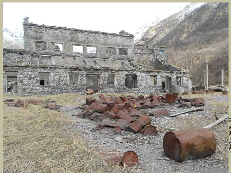
Photo 5: Arsenic-containing drums and debris from the old factory, Tsana 3
