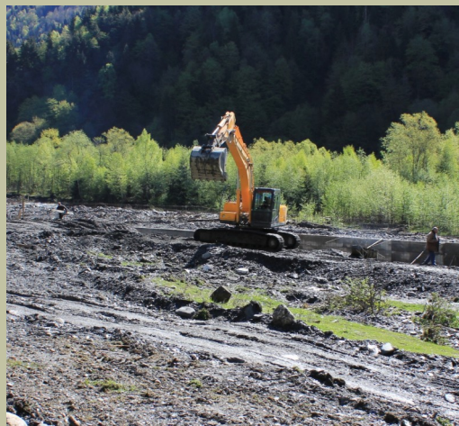
Photo 7: Construction of a protective dyke - Tsana 1
