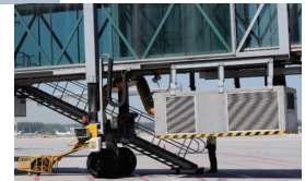
Fig. 4.2 Efficient Ground Bridge Loaded Power Units replaces Auxiliary Power Units
