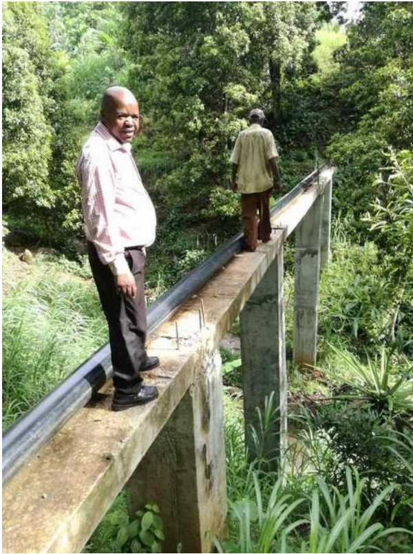
River crossing for the partially rehabilitated transmission main, Nieumakélé
