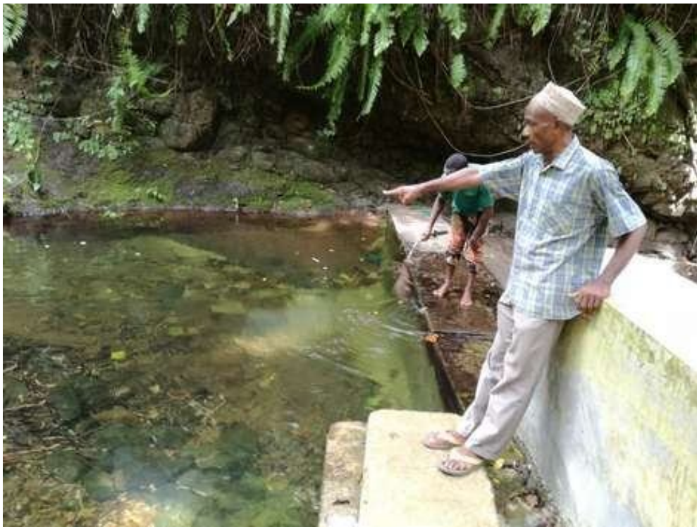
Rehabilitated intake, Lingoni-Hoani water supply scheme
