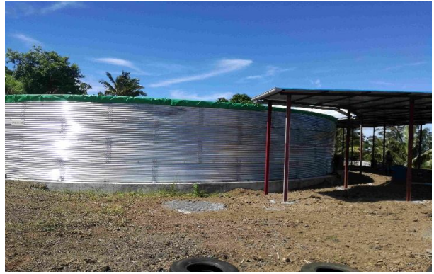
Water harvesting Reservoir, Bandas. (CRCC financed)
