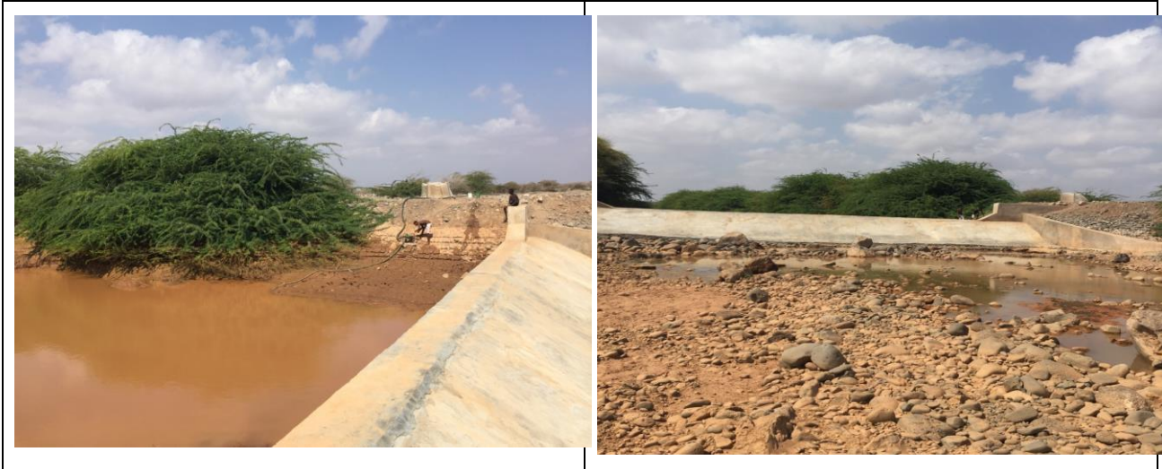
Figure 7: Photographs of Upstream and Downstream of a Micro Dam in Damerjog
