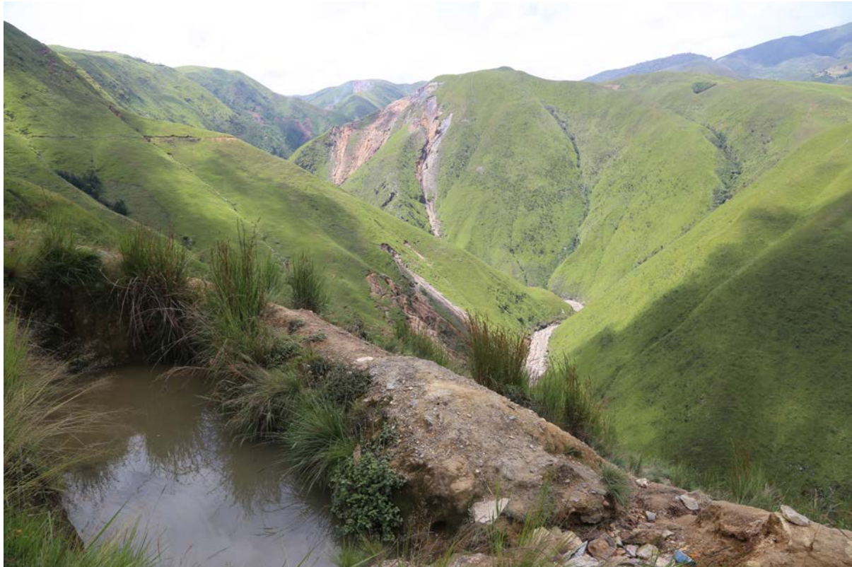
Photo 28: Water collection pits located above the Butuzi mine site increase infiltration into landslide initiation zones
