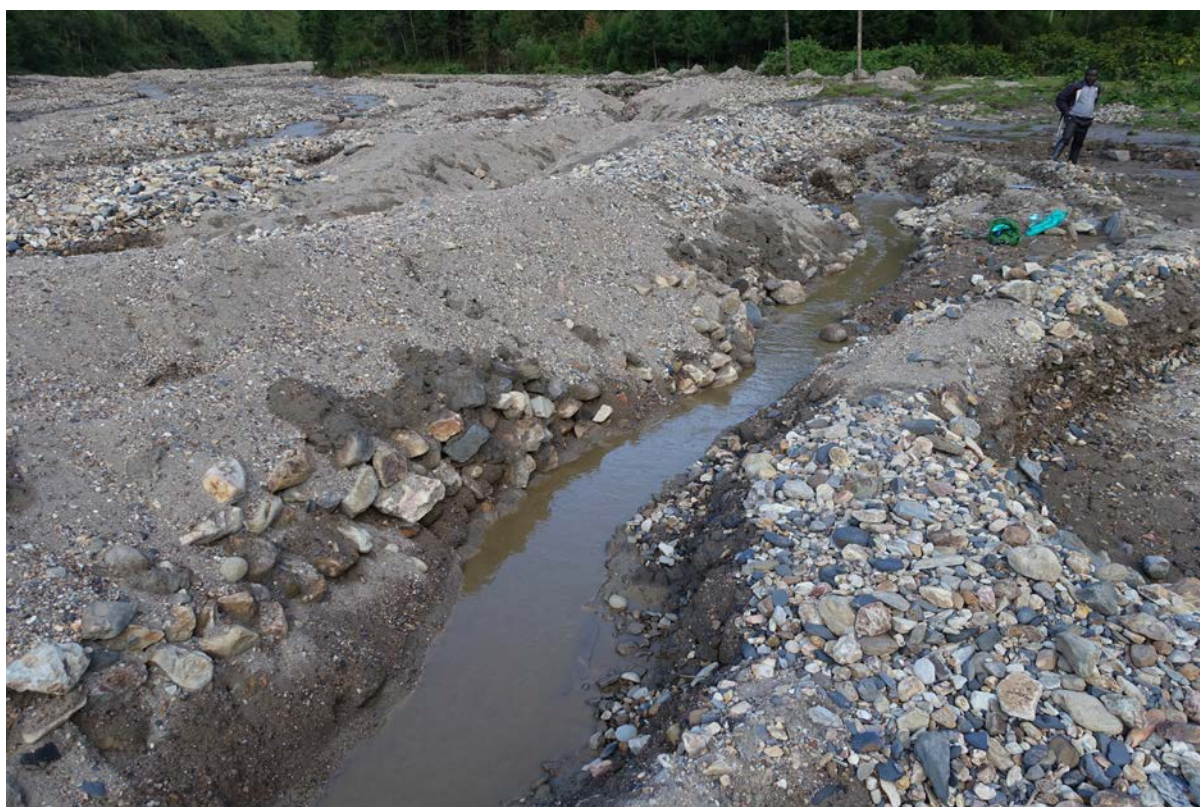
Photo 8: Wall and channel structure of heavily worked river bed
