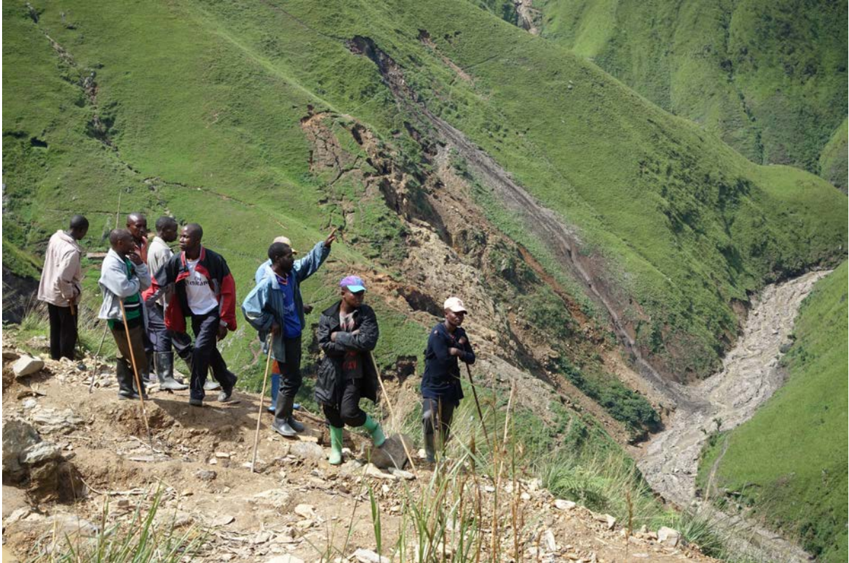
Photo 7: Note the web of cracks in the copper mine on the adjacent slope, and the grey waste rock dump slide stretching half way across the riverbed. Sinuous patterns created by walled channels built by the alluvial miners can also be made out below
