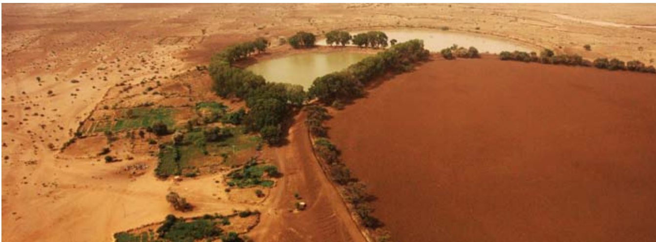
The heavily silted Golo Reservoir in El Fasher. To control silting in the reservoirs like Golo, erosion control is needed in the upper reaches of the wadi. This requires a holistic approach to catchment management.
