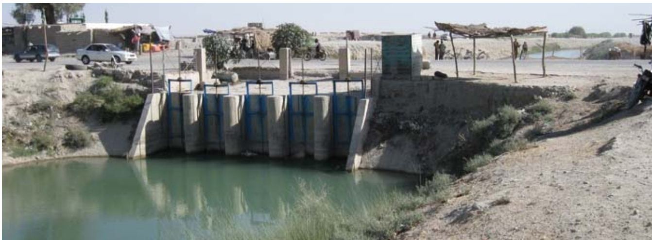
Work on the Shamalan Canal is coordinated under the Helmand and Arghanadab Valley Authority. The canal is being rehabilitated as part of the broader post conflict reconstruction effort in Afghanistan.
