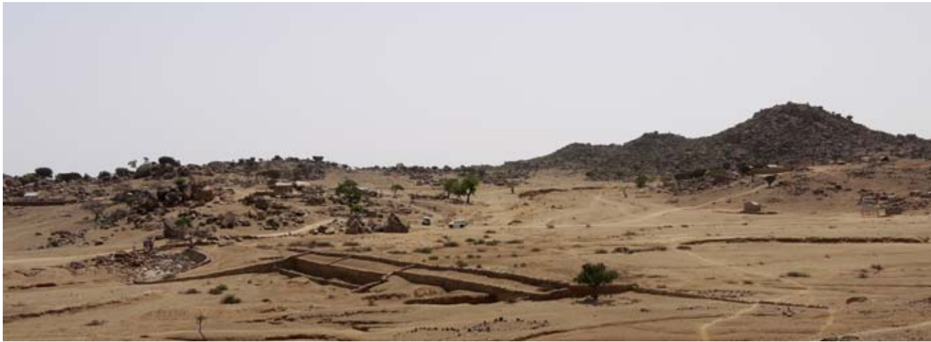
At Ar Keweit, Red Sea State, sand dams, like this one, are used to reduce soil erosion and improve agricultural production in the area. It is part of a larger community based catchment management approach.
