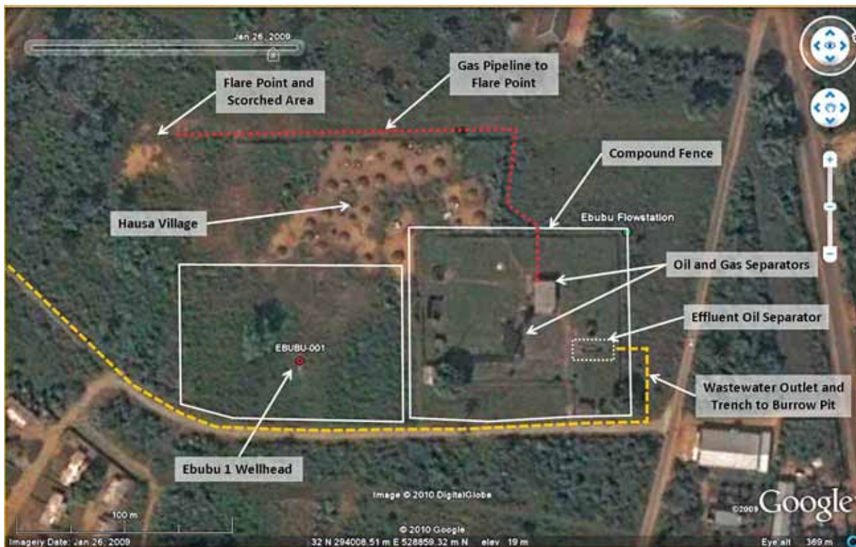
Typical flow station and associated infrastructure (Ebubu Ejama, Eleme LGA)
