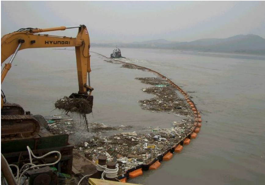
Figure 30. Trash boom at the Han River during the flood season.
