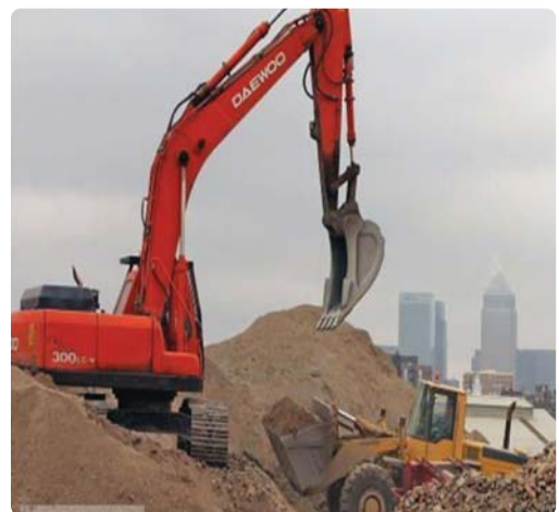
Excavator at work
