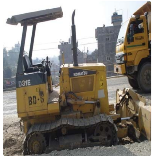
Bulldozer at work
