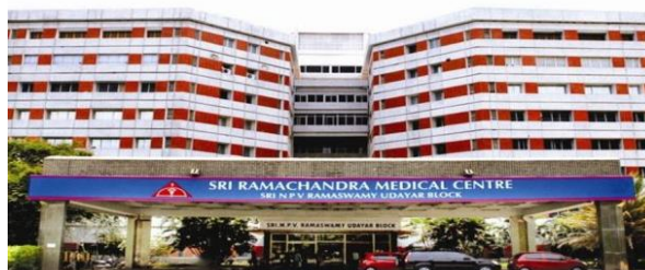
SRI RAMACHANDRA MEDICAL CENTRE, CHENNAI, INDIA
