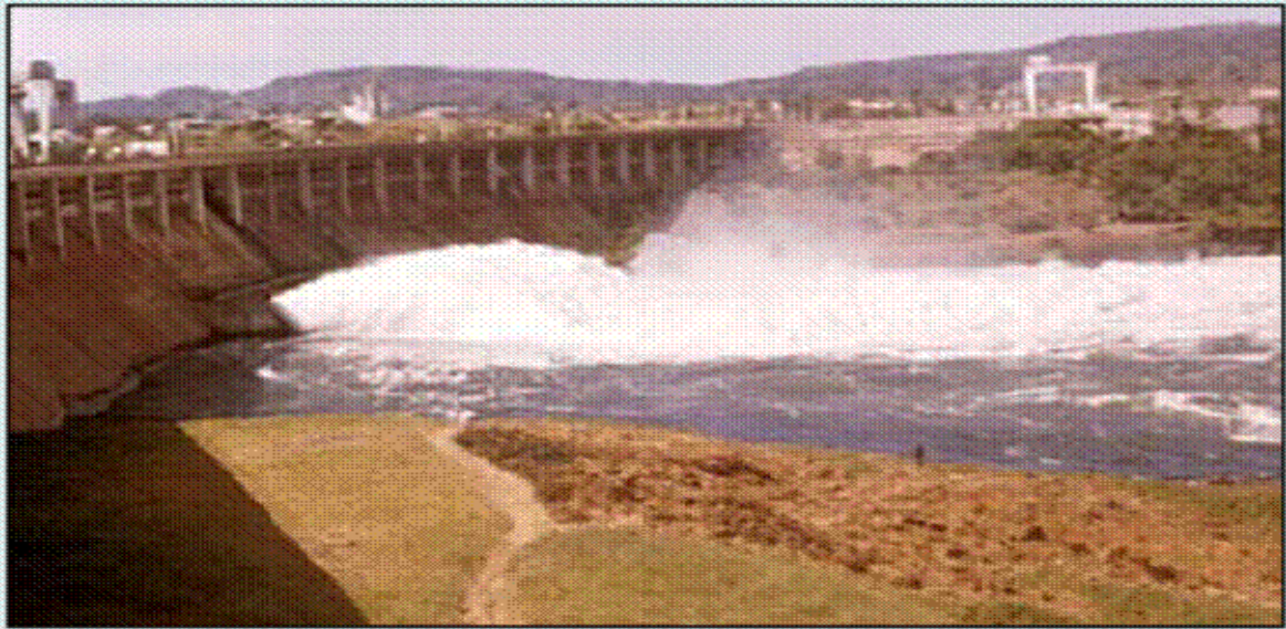
Photo 3: Nalubaale Power Station (Owen Falls Dam)
