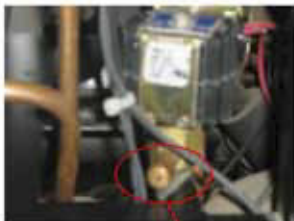
Air out port controlled by Solenoid Valve
