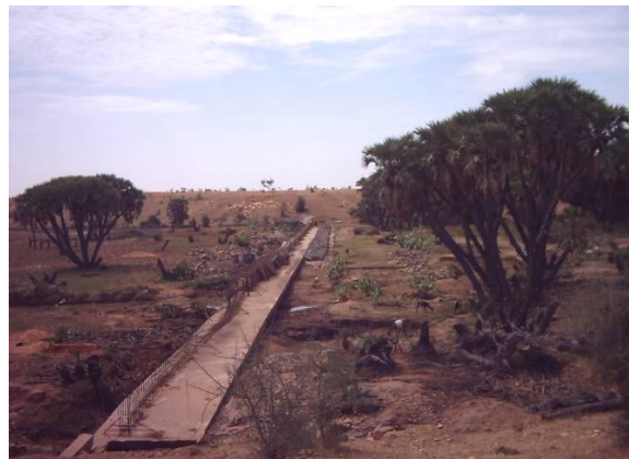
Photo 11. Barrage Oued Niakhlée (15° 53' 42" N, 11° 32' 04" O) (ECODEV, 2009).
