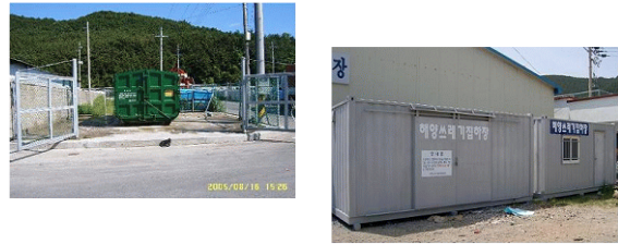
The picture of depositaries of marine wastes
