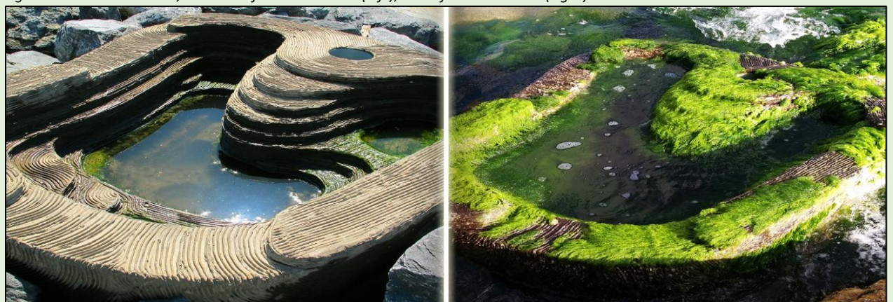
Figure 3. Tidepool Armor, minutes after installation (left); and after 12 months (right).
