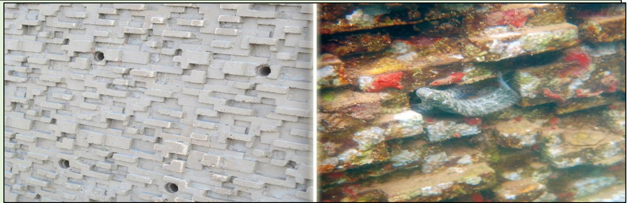
Figure 1. Eco Seawall, before installation (left); and after 12 months (right).
