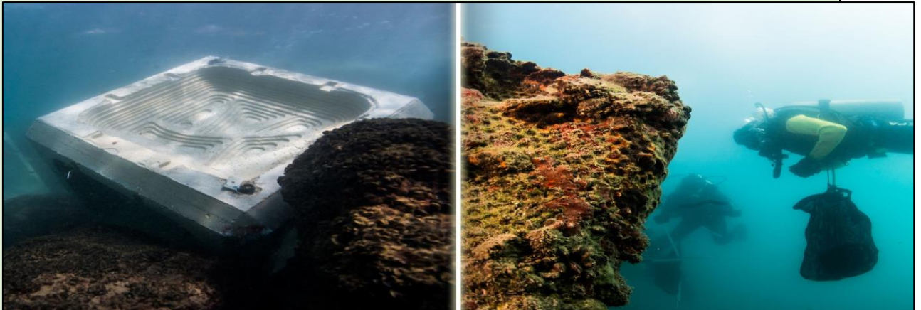
Figure 2. Eco Armor Block, minutes after installation (left); and after 24 months (right).
