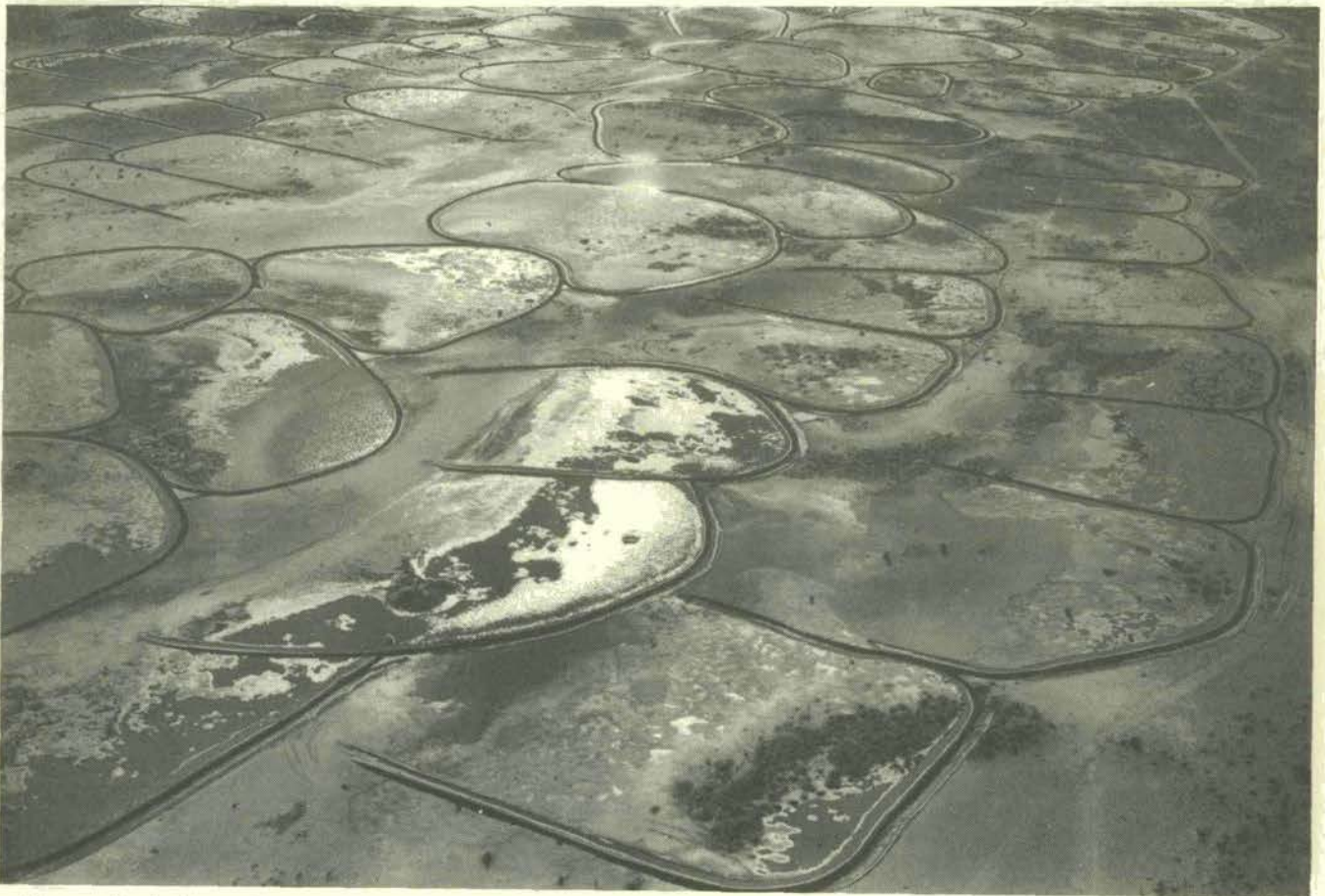
Water ponding banks on a bare scalded area north of Nyngan, 134 km. east of Cobar, New South Wales. Yields of forage from the ponds have repaid their construction cost many fold.
