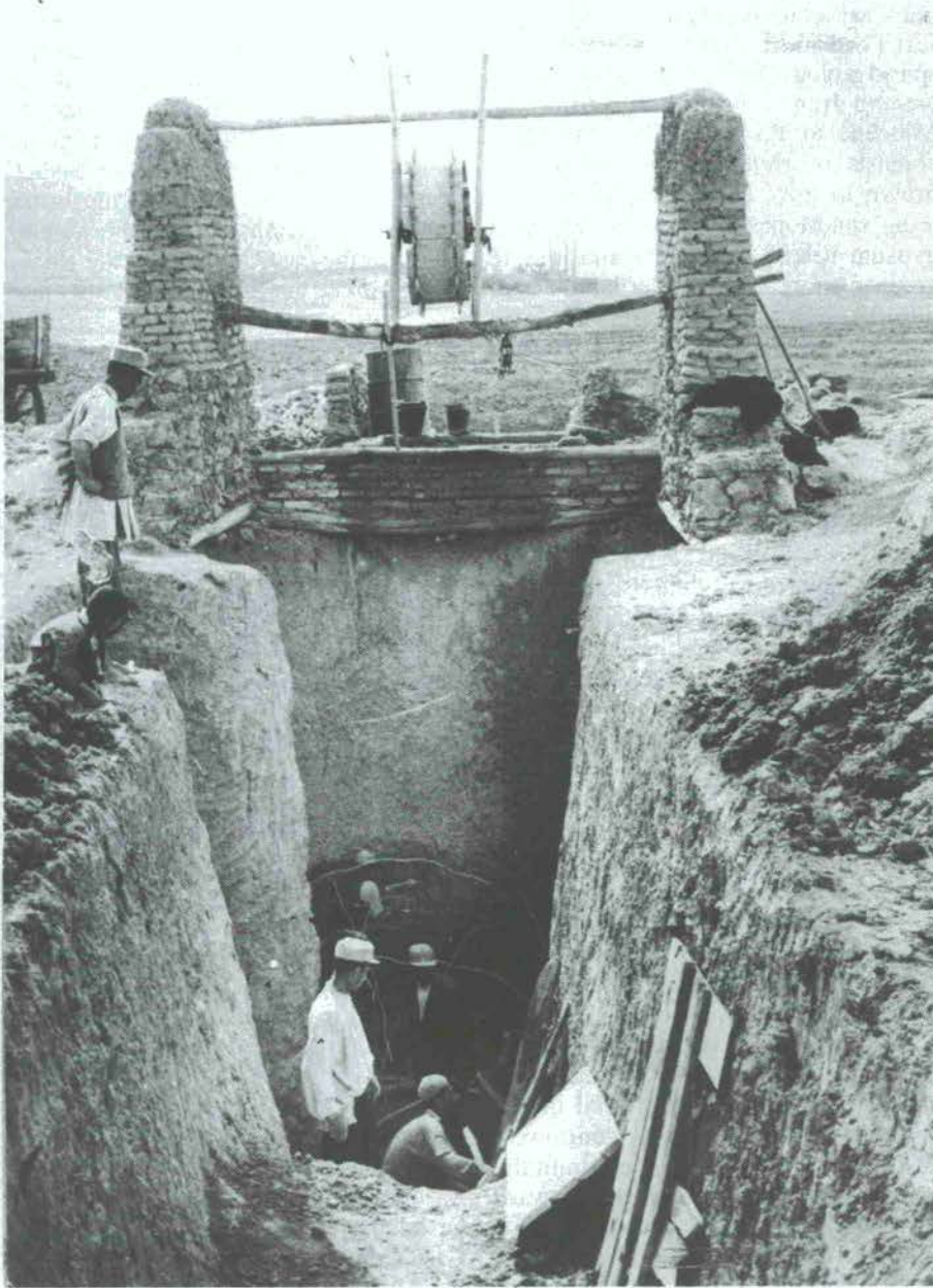
The "qanat" —an ancient irrigation system used in certain arid regions of Iran. It is a horizontal well with canals dug deep into the slope, leading from one qanat to another in order to avoid evaporation. They are fed both by rain and ground water. Photo: Paul Almasy
