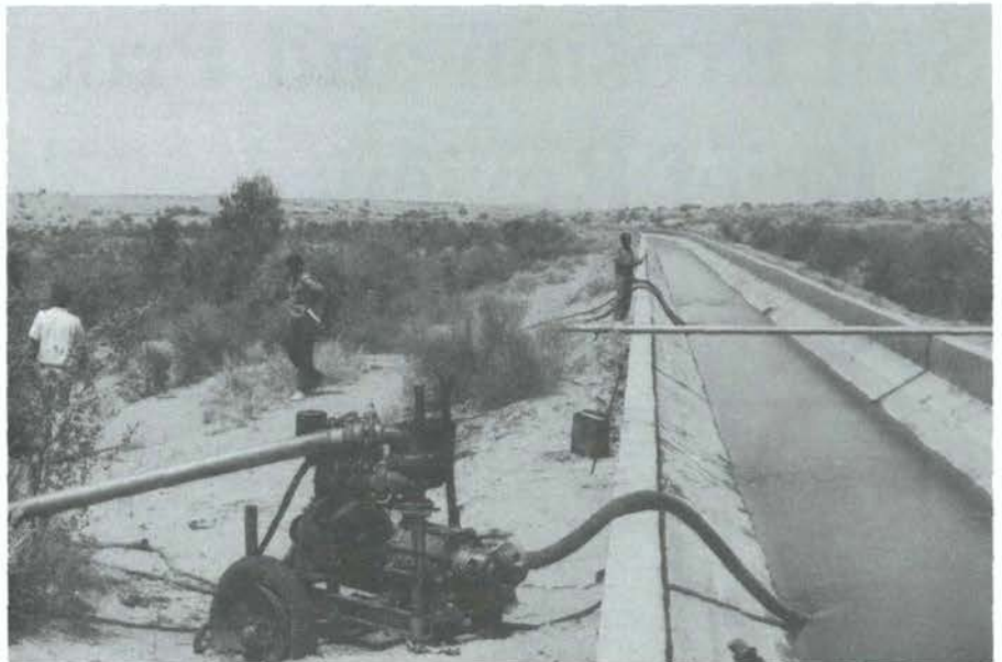
A distributary of the Indira Gandhi canal at Bikaner. The water is lifted and siphoned for afforestation on both sides. Photo: R.K. Sinha.
