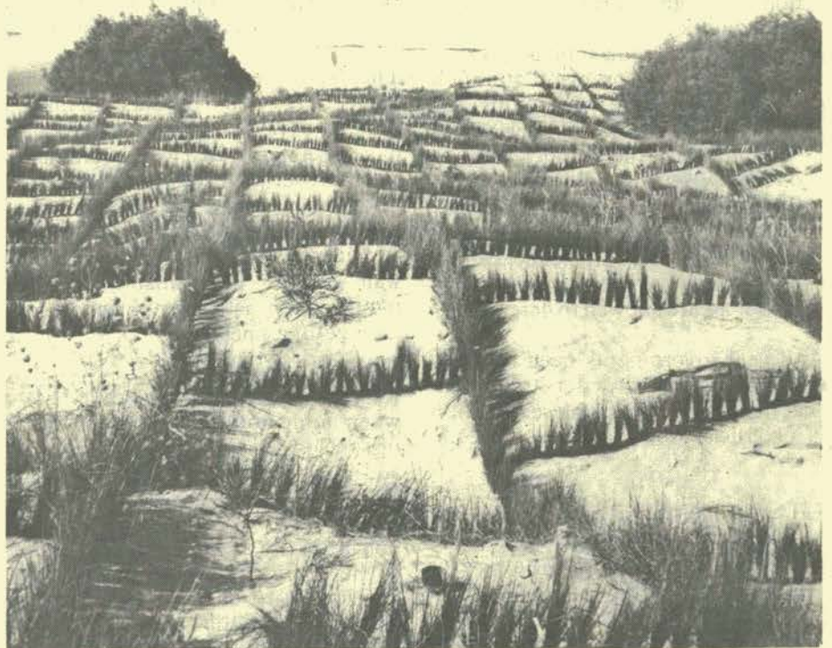
Sand dune fixation projects, such as this one in Libya, serve to prevent the covering of productive lands by moving sand dunes. (UN)
