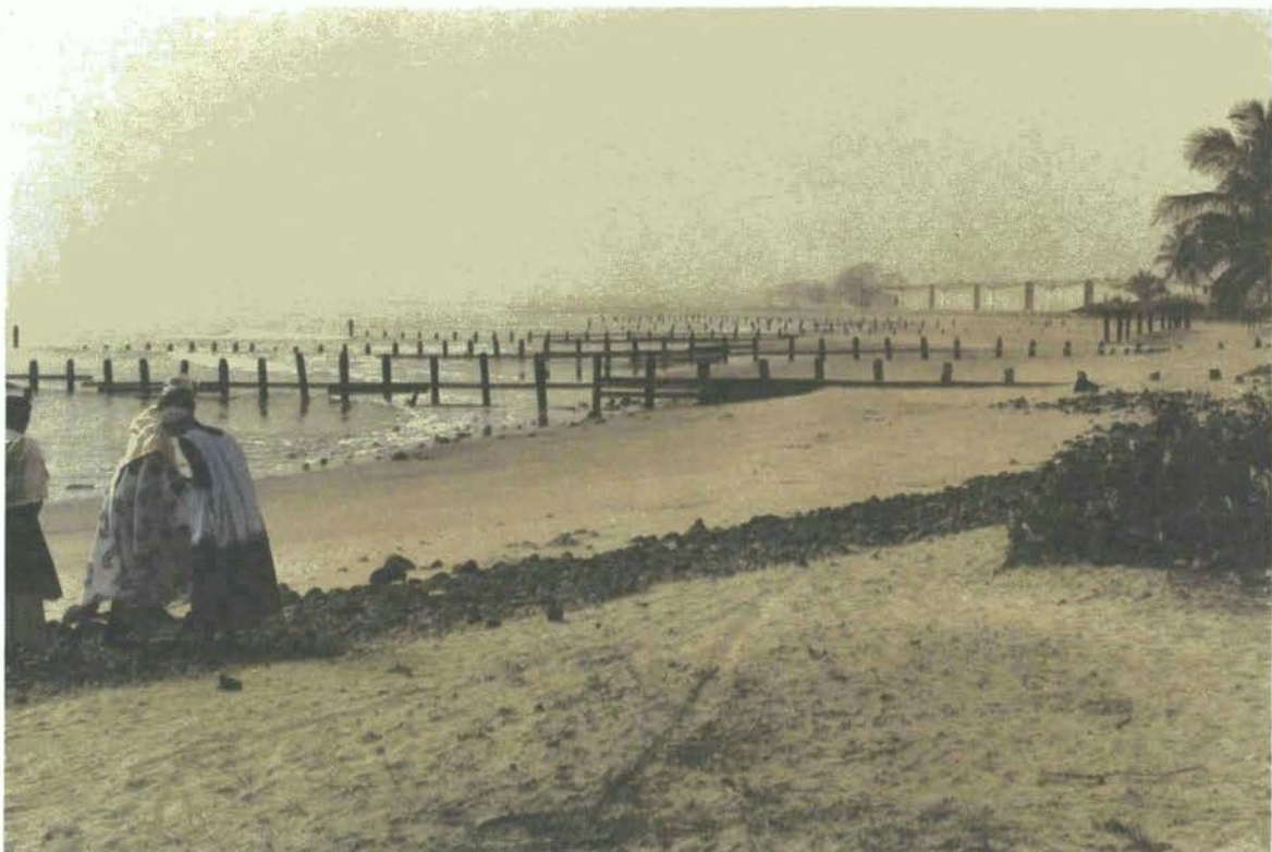
Fig. 5.3. - Beach protection at Cape St. Mary (Gambia) by using wooden groins. (Quélenec, 1988).
