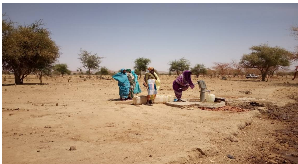
Figure 3. Water Pump in Ashamara, WD
