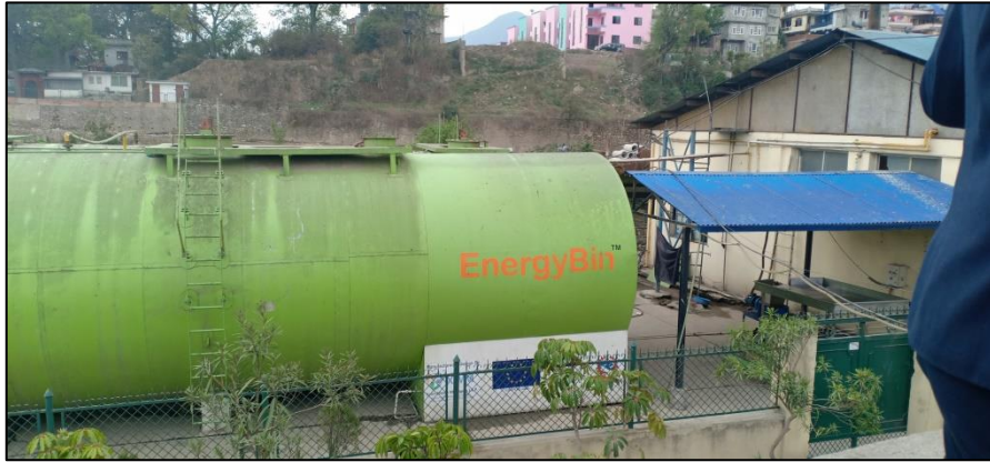
Photo : Waste to Energy Plant of KMC which generated 14 KW of electricity every day from 3 tons of waste. According to KMC, It is currently under repair.
