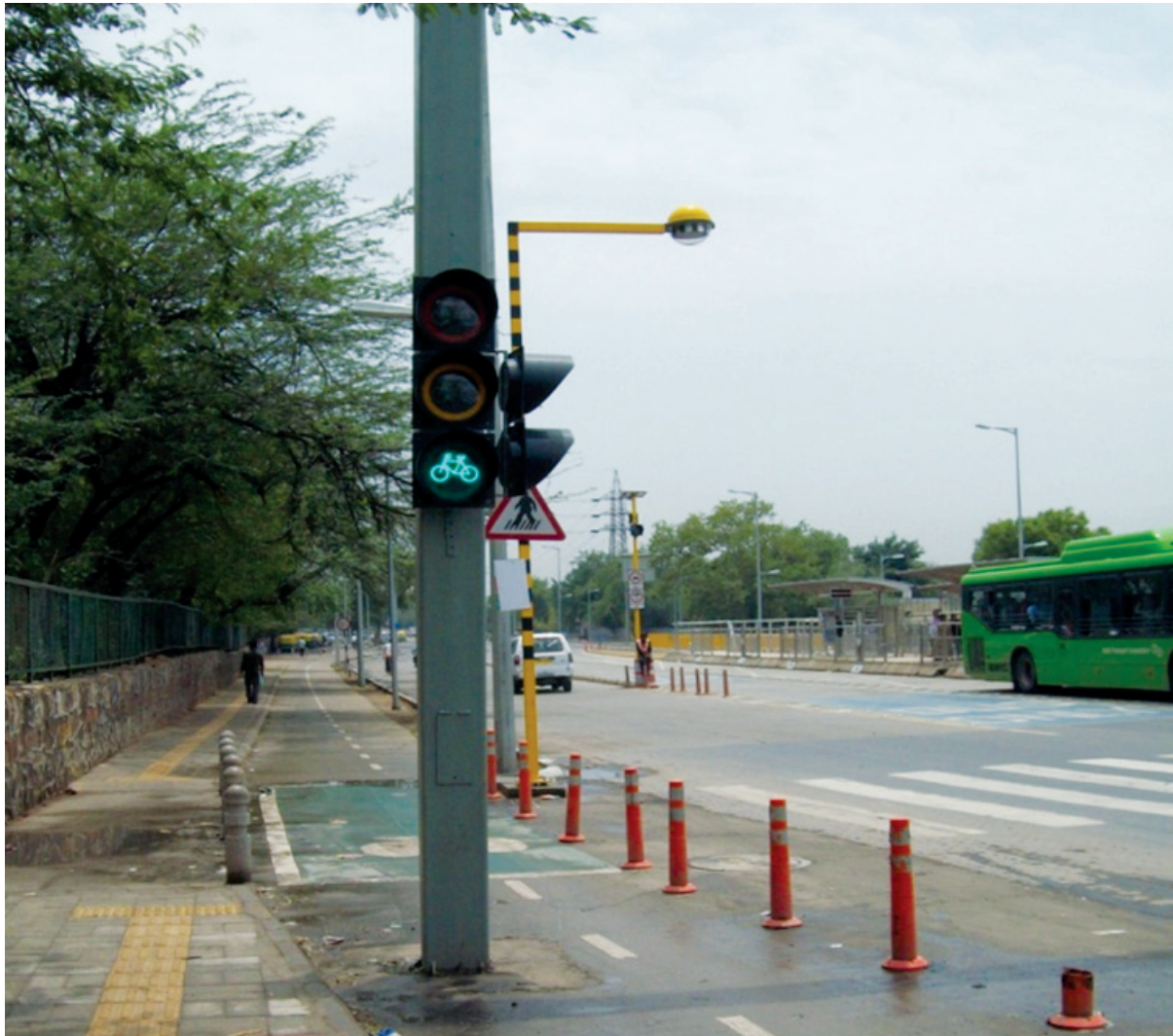
Figure 13: Special traffic signal for NMT on Delhi BRT corridor
