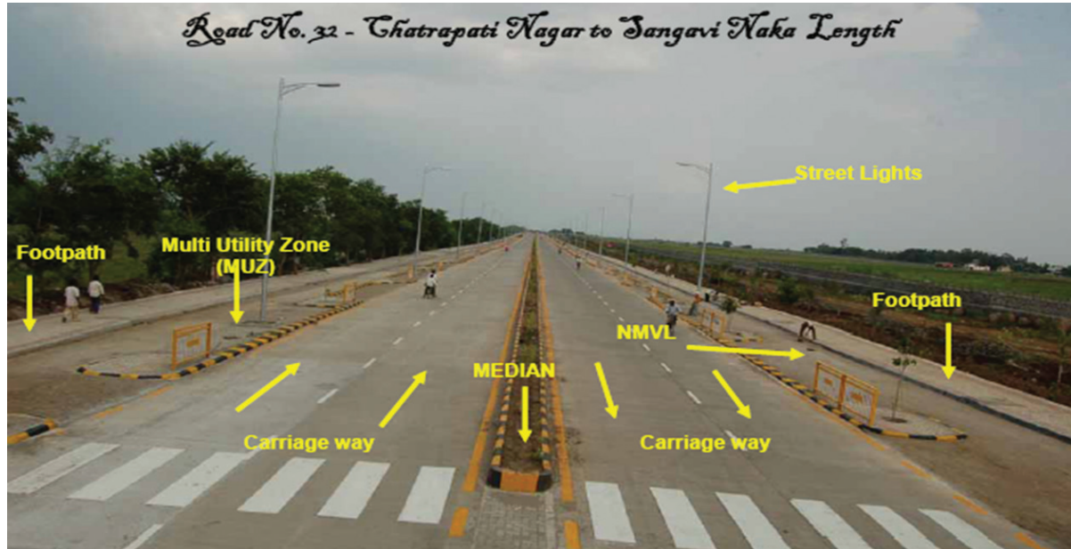
Figure 8: Upgraded streets of Nanded
