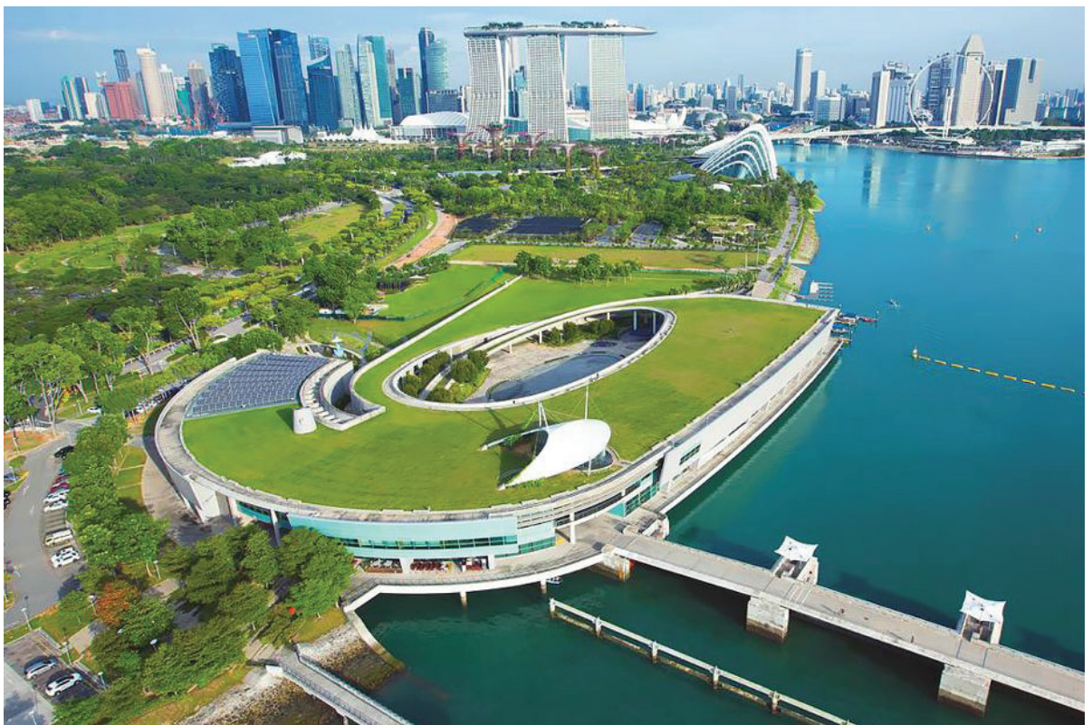
The Green Roof at Marina Barrage
