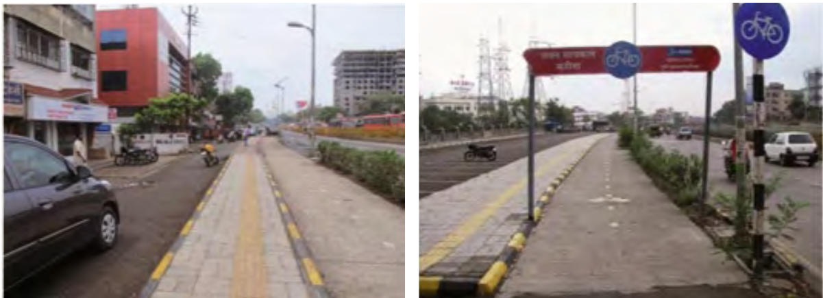
Figure 8.2: NMT lane along the BRTS corridor in Pune
