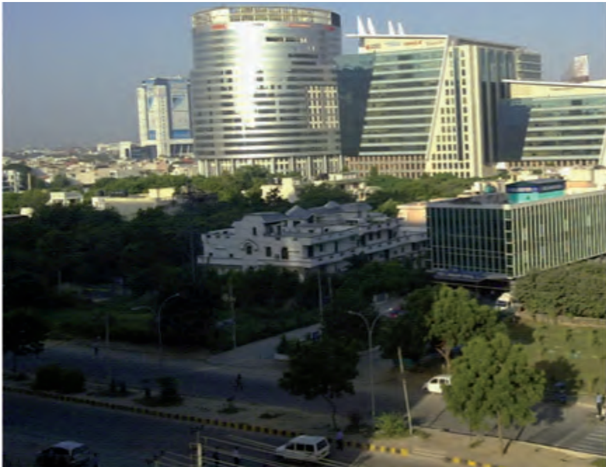
Figure 7.1: A newly developed area in Gurgaon with no footpaths
