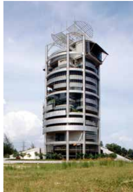
Figure 8a • A MODERN BUILDING WITH PASSIVE DESIGN ELEMENTS IN SELANGOR DARUL EHSAN, MALAYSIA (Aga Khan Development Network, 2016)
